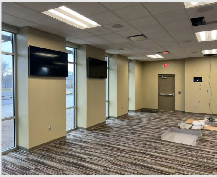
Audio and visual installs are occurring in the Community Room.
