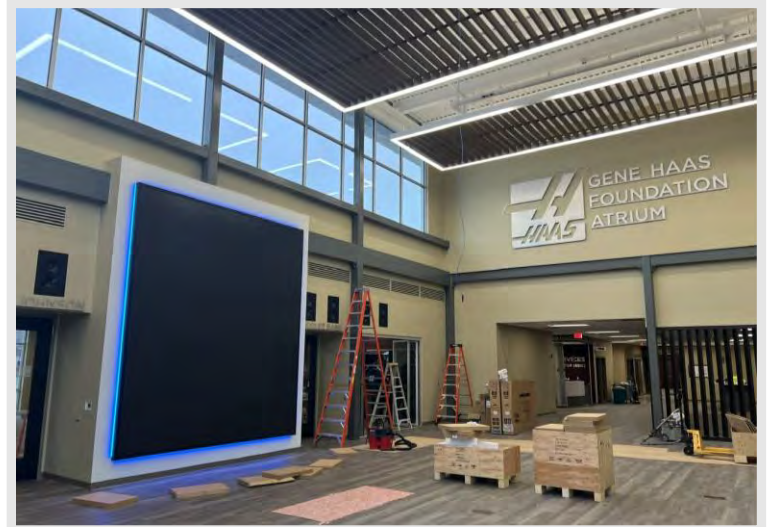
The displays for the atrium's video wall are installed.
