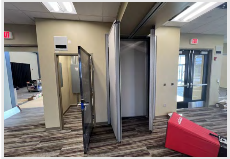
The operable partition was installed in the Community Room.
