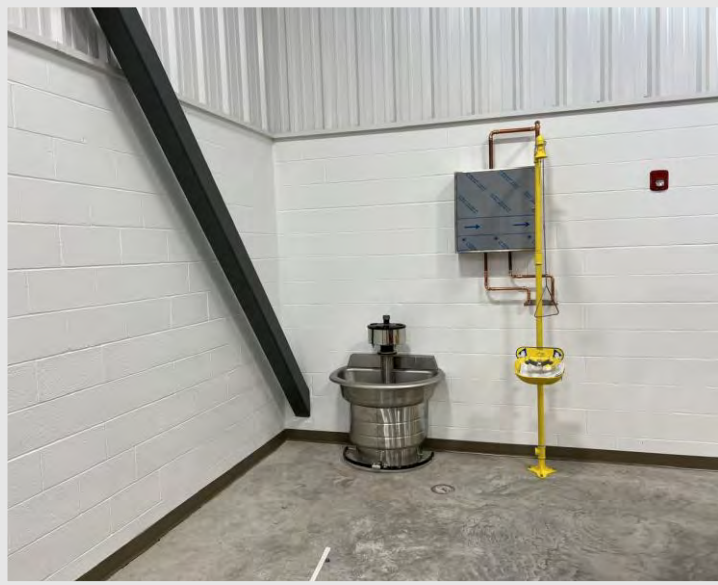
Plumbing fixtures were installed in the labs in the past week.
