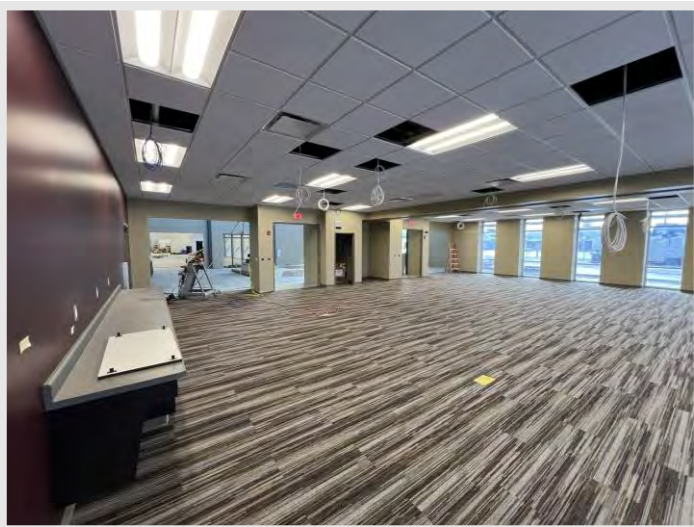
Flooring installation has taken place in the Community Room.
