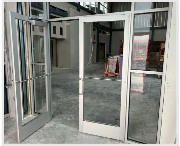
Aluminum storefront door installation is taking place at entrances.
