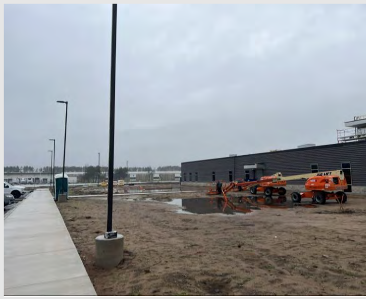
Exterior light poles have been set throughout the project site.
