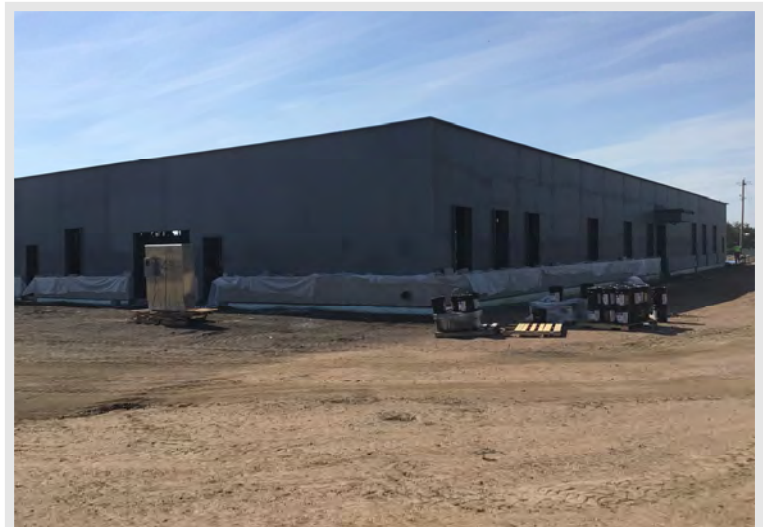
Split face wainscoting has finished around the exterior of the building.
