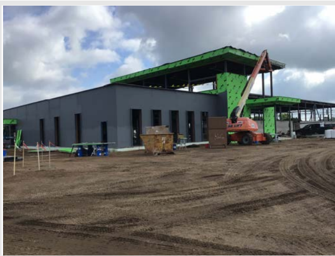
Air vapor barrier is following the exterior sheathing to get one step closer to weathertight.
